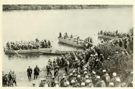
French Army: pontoons used for ferrying troops across a river or for constructing a floating bridge.
