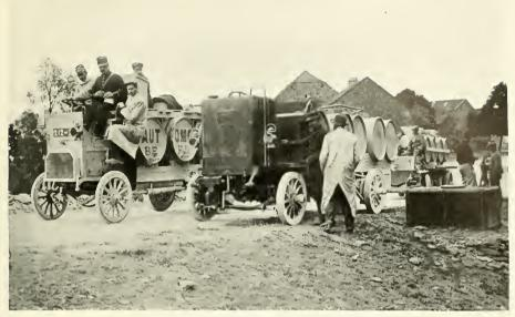
French tank motor-trucks for carrying pure water.
